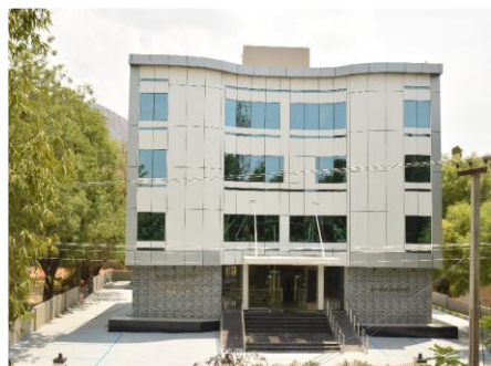
Pratap V. Reddy Feed Analysis Lab Building
